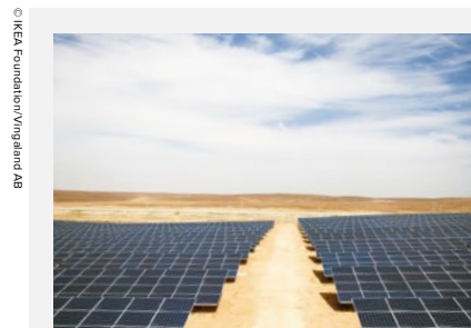
Azraq refugee camp's new solar farm stretches out into the desert.
